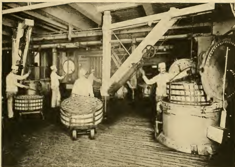
FIG. 66.—Commercial retorts where steam is piped in from the boiler. (Heinz Company.)
